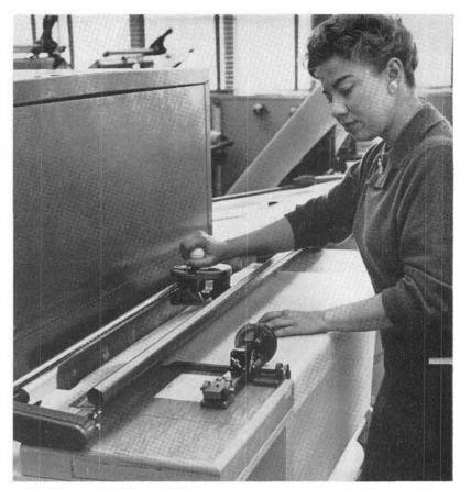
HANDY CUTTING DEVICE is demonstrated here by Vonna Burroughs to cut and measure plastic drawing material used by Sandia Lab draftsmen. The combinaton of cutter, counter, storage cabinet, and rack was designed by Daniel J. Alvino, Gabriel C. Beatrice, and Donald N. Cox of Division 4412. Assembled from modified readily-available parts, it saves time, prevents waste.
